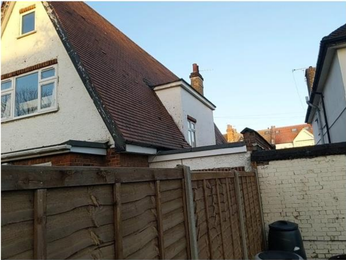
View of rear and side of no. 18
