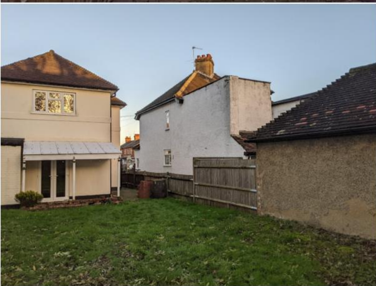
Rear of host property view of no.14
