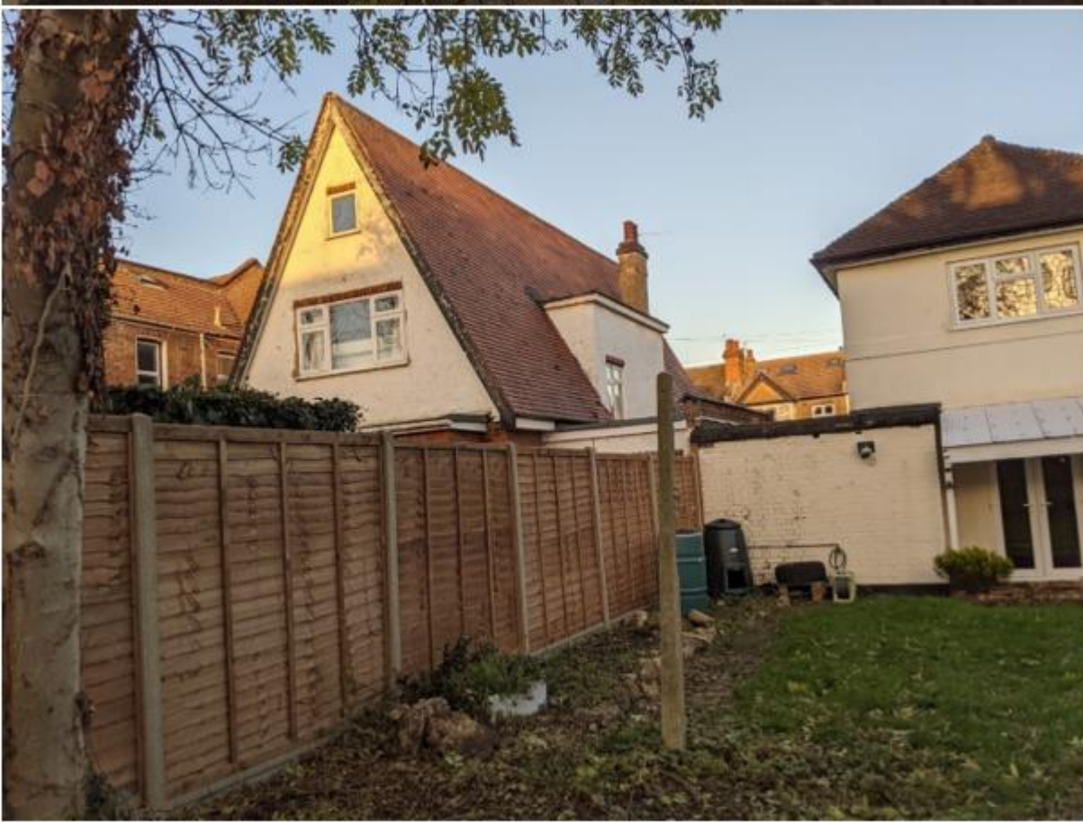
Rear of the site view of no.18
